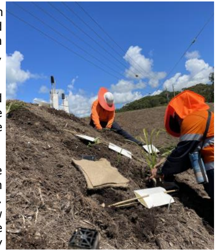
Above: Planting on the slopes with plant guard kits.
