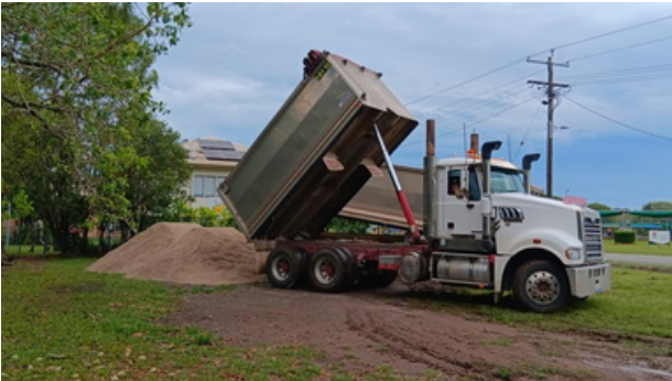
Above: Harris Haulin delivering material for the walking track upgrades
